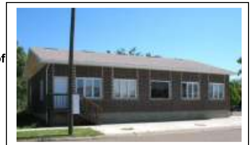
South side of building
